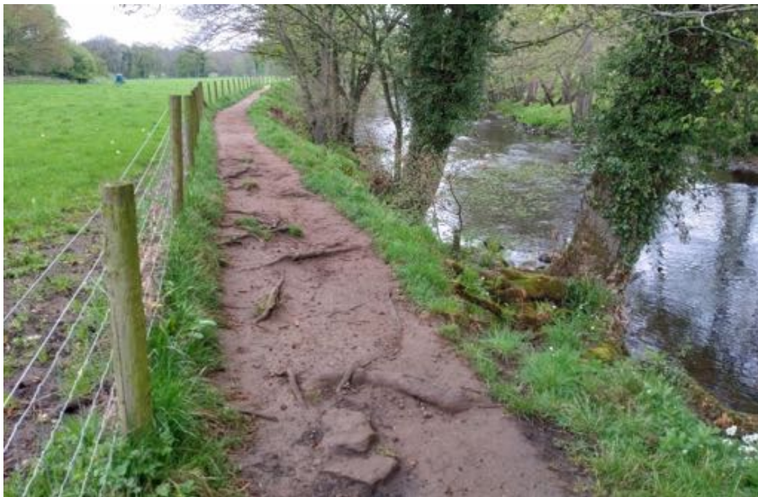
Fig 2a. 54.034378, -1.6867578 at the d/s end of Reach 1 where the proposed greenway joins from Station Rd in Darley and runs parallel to the river. The existing footpath was typically <1m width, heavily used, and the footfall keeping the path free from plant growth has exposed the roots of mature trees within the bank. Formalising the greenway here will irreparably damage those trees. Note, there was little evidence of self-set regeneration of trees under the current scenario (so even less under the proposal), primarily because there was insufficient space in the riparian zone ie between the path edge and the bank toe (waterline).
