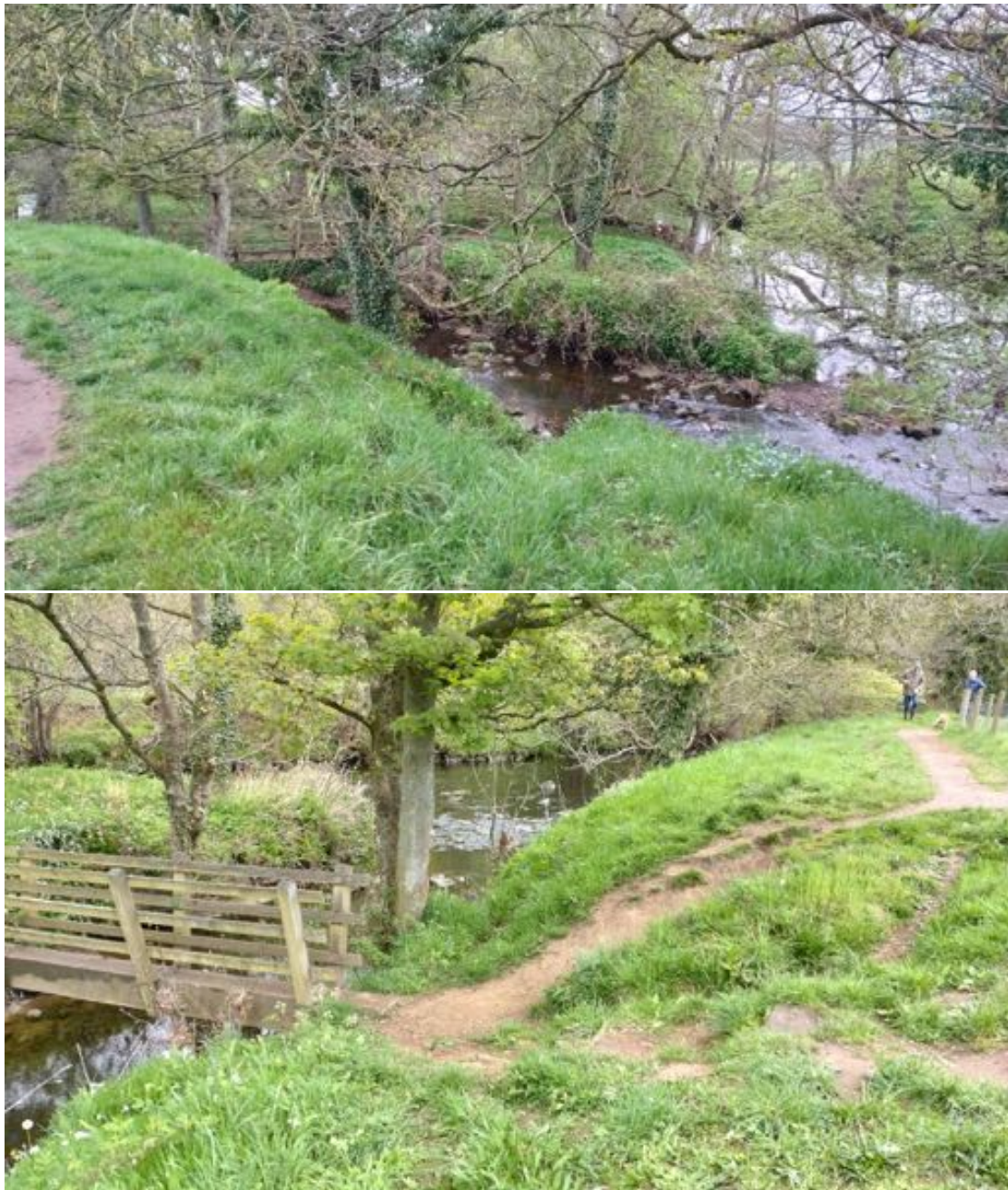
Fig 3. 54.03637, -1.6891176: The confluence of Darley Beck with the mainstem Nidd and existing footbridge. The area is prone to frequent inundation during spate flow when water from Darley Beck backs up against a typically much higher Nidd. Tree cover and diversity was good, but the understorey was compromised in various places by footfall accessing the beck. These desire lines, generally created by dogs, can lead to further erosion and ingress of fine sediment.
