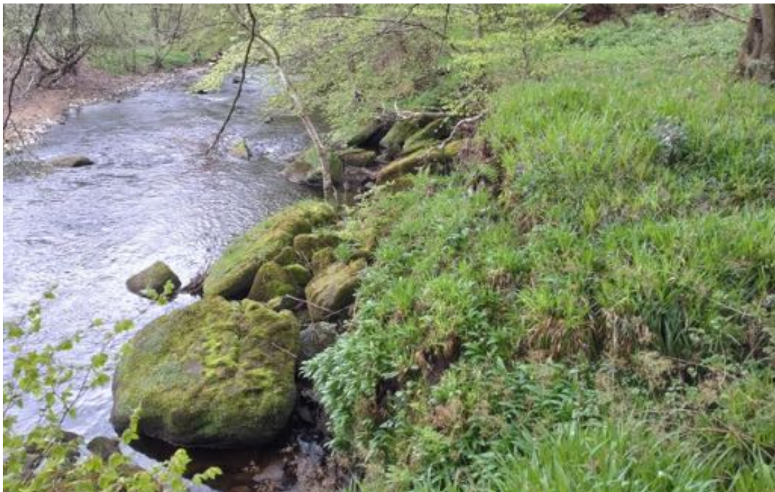
Fig 8. 53.927199, -1.7678501. Large boulder revetment, historically used to protect the right bank from artificially accelerated flows caused by routing the river perpendicularly across the valley and under the former railway line.
