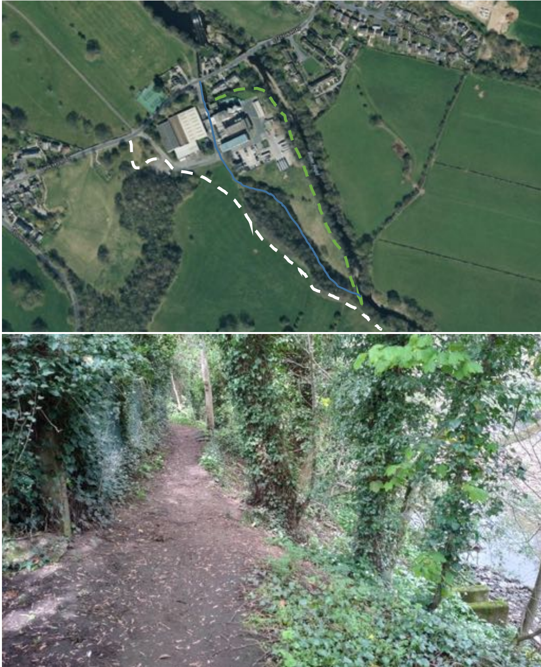
Fig 12. 54.031850, -1.6280485: The feed factory at Birstwith presents a dilemma. It is a former mill and sited on an island created by the mill leat (blue line) being taken off from the Nidd at the weir u/s of Birstwith Bridge.
